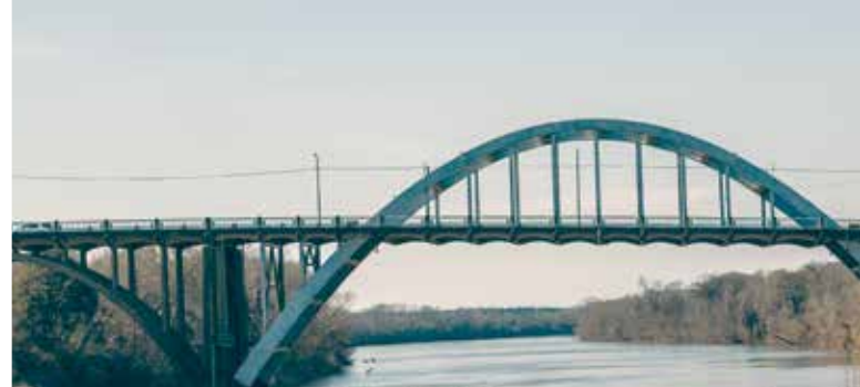
Selma Bridge Over Alabama River
