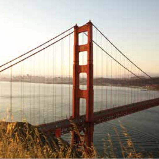
Golden Gate Bridge
